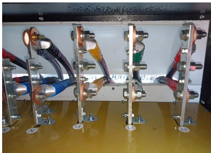
Figure 6.18 Diagram of junction box wiring
