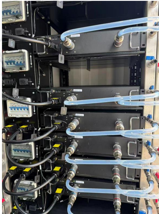
Figure 6.15 U-type Server Piping Connection Diagram
